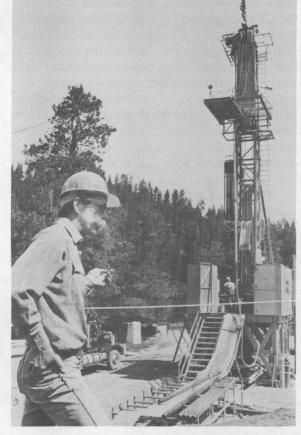
AS PETE LYSNE (6252) explains to a site visitor (out of camera range), the 50-ton drill rig sits 12 feet above grade (note rig wheels in large photo). The extra height permitted installation of main BOP (blow-out prevention) stack, a series of valves that can shut off the flow of fluids or gases to the surface whether or not a drill string is in the corehole.
